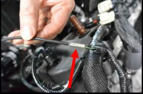
39. Install the supplied ground wire with eyelet using the 5mm flanged nut to the factory valve cover stud. Secure using an 6mm socket.
